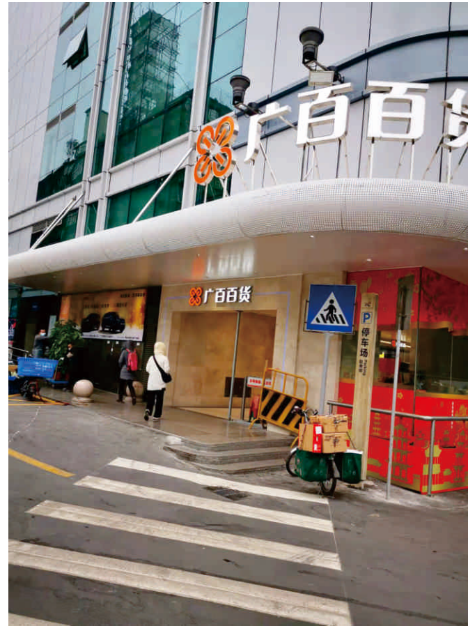
Guangzhou Beijing Road Guangbai Department Store (curved punched mesh plate)
