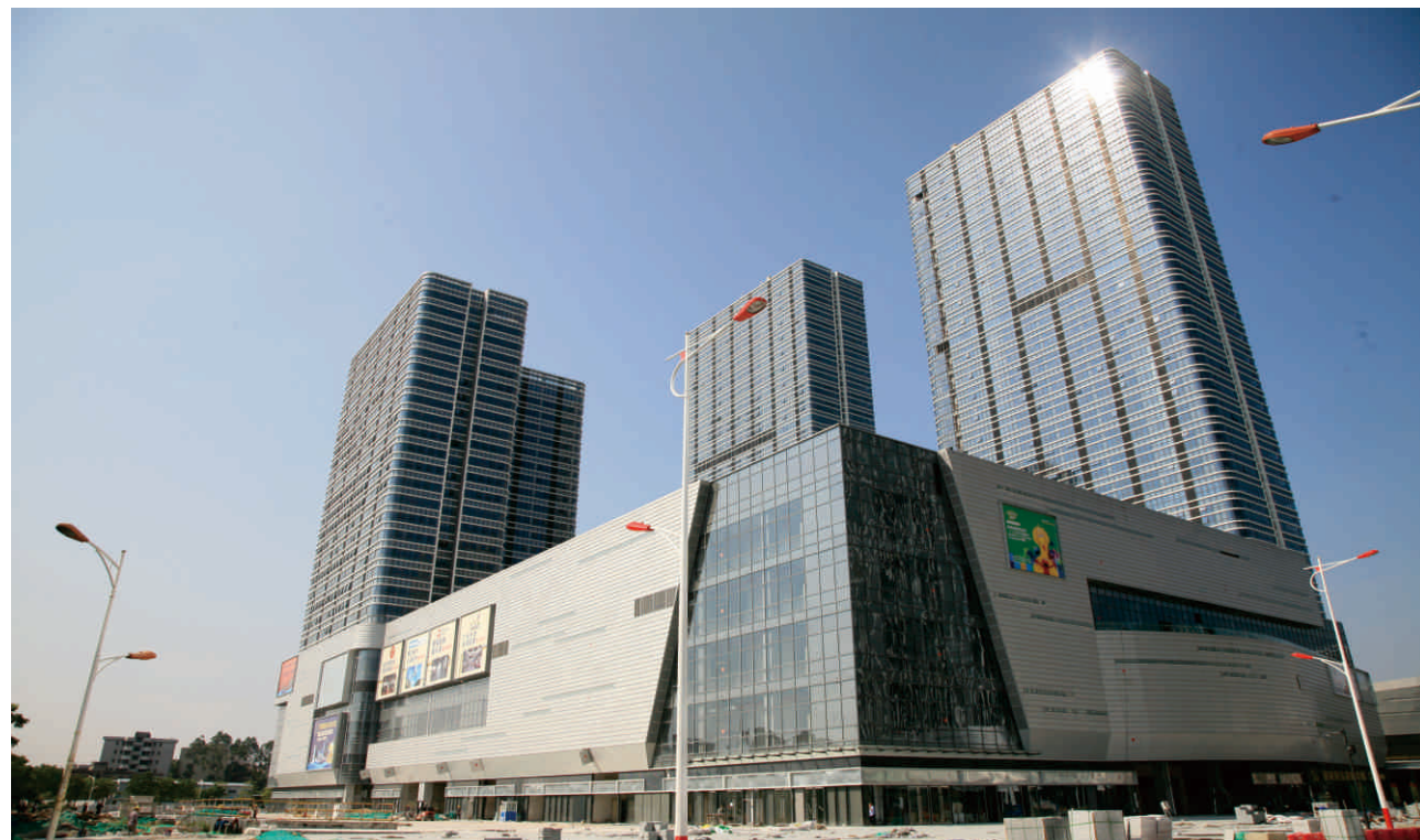
Foshan Starport International Plaza
