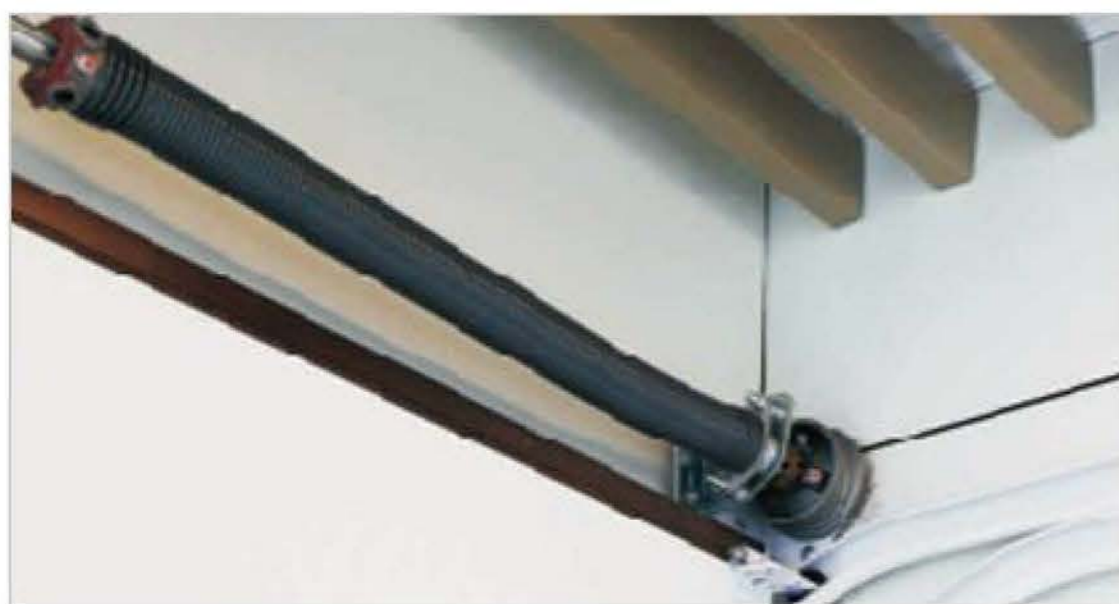
DELICATE TORSION SPRING BALANCE SYSTEM
